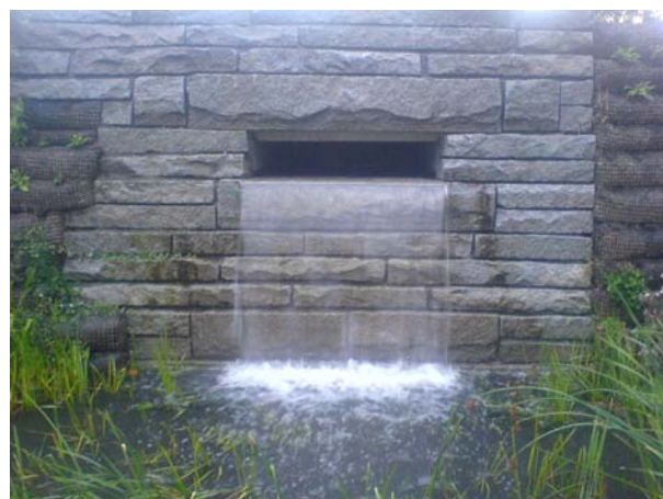
1 Water enters through the Upper Cascade Waterfall
