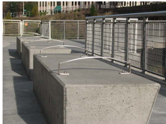
3 Cast-in-place concrete benches
