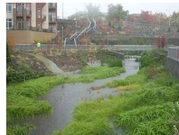
3 Water in the Low Flow Channel
