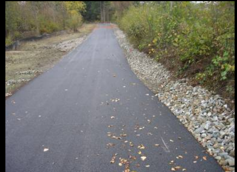
Porous Asphalt Drive, Pierce County
