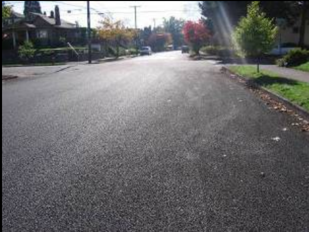
N. Gay Ave, Portland. Porous Asphalt Concrete (2005 - 8" porous AC over 6" Subbase)
